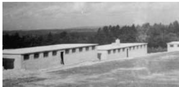
Detention barracks Erie Camp in 1941 under construction
