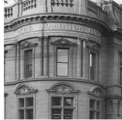
The Dominion Bank of Canada
